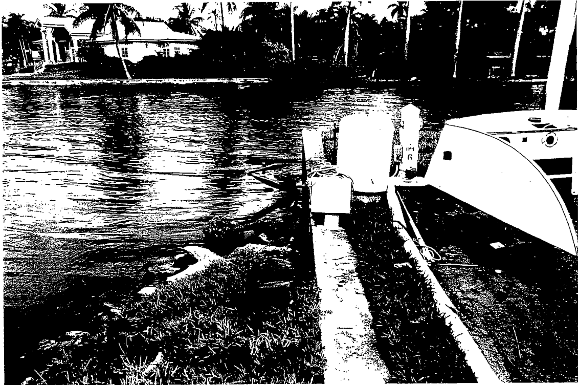
Looking North @ West Subject Property Boundary Along West Side of Concrete Bulkhead
